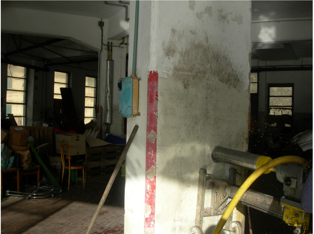
C8 – Pilastro 3° piano
